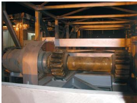
Coke pusher drive
