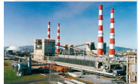
Coke oven plant
