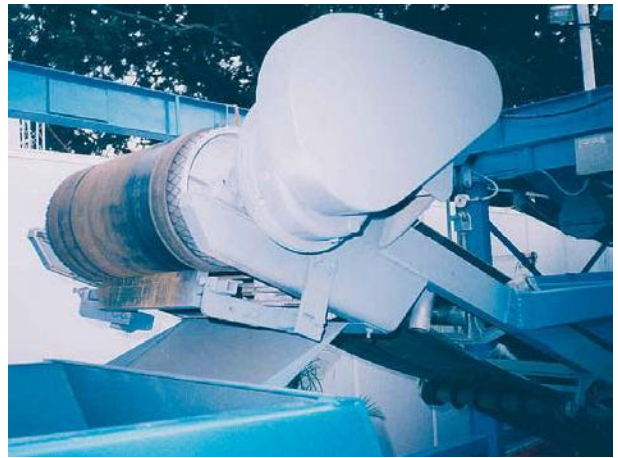
Feed conveyor in batching plant
