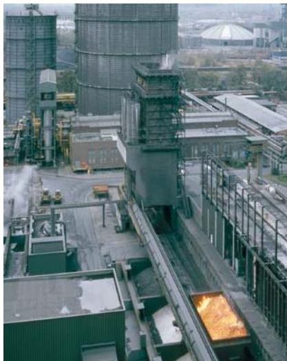
Quenched coke pusher
