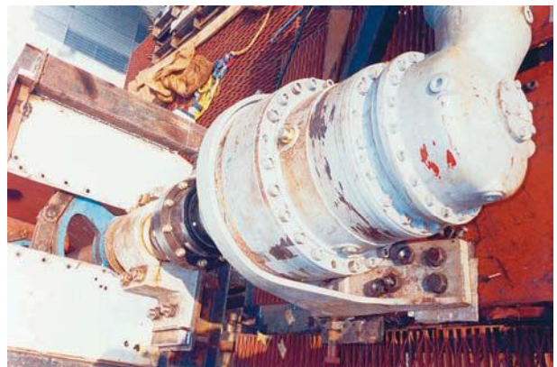
Bagasse carrier drive in sugar plant
