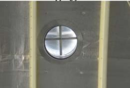
• Installation at areas away from ridge / sheet overlapping joint line - flashing sheet required
